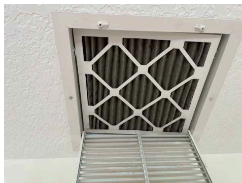
Rear right bedroom ceiling
