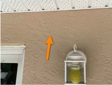
Rear side above sliding glass door
