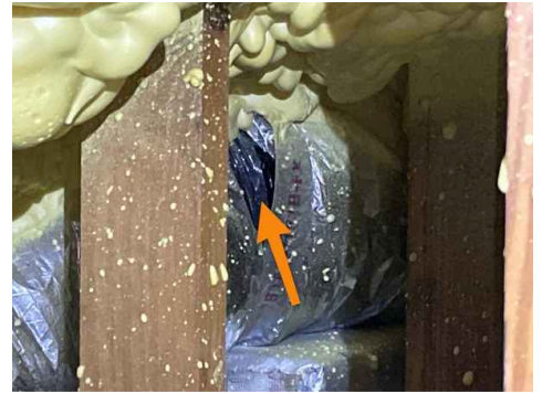
Right side of attic above air handler
