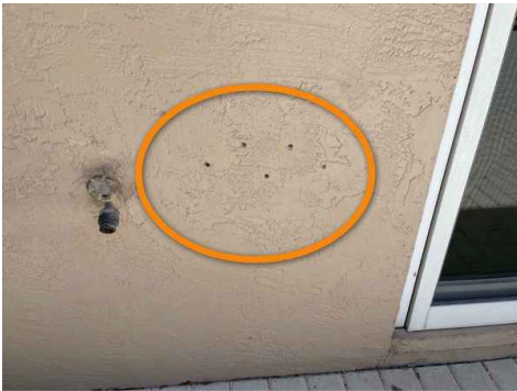
Rear side to right of sliding glass door
