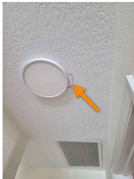
Hallway by kitchen
