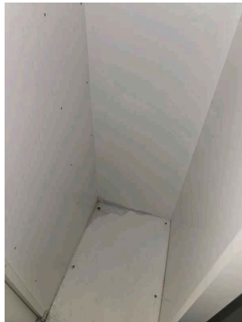
Laundry room utility closet
