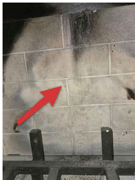
Firebox cracked
